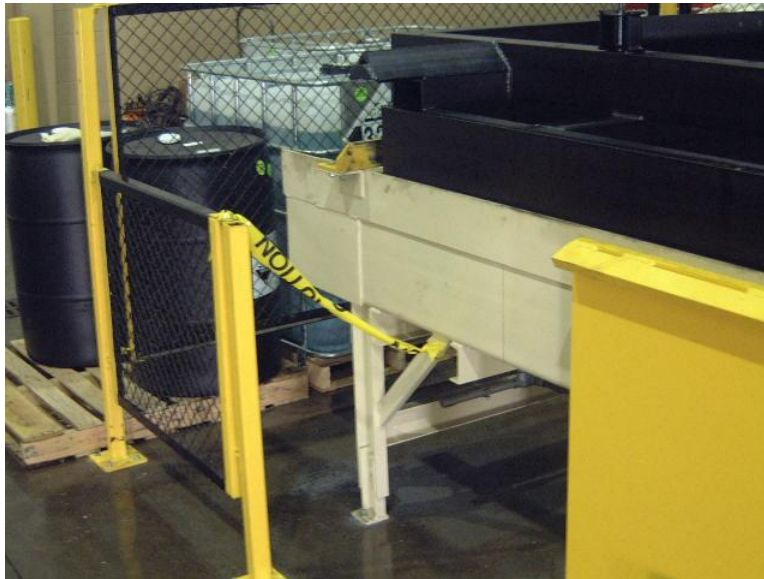
Figure 4 Poor execution creates waste and potential liability
