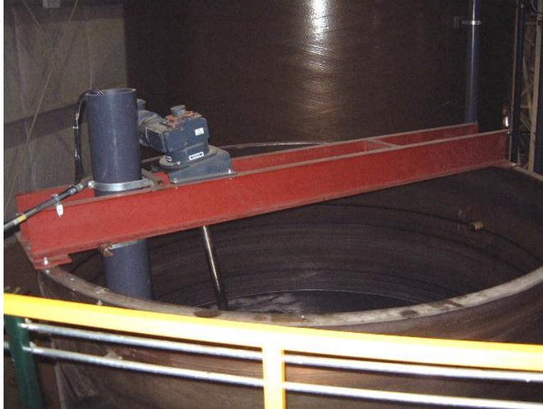
Figure 5 Motor and impellor without access
